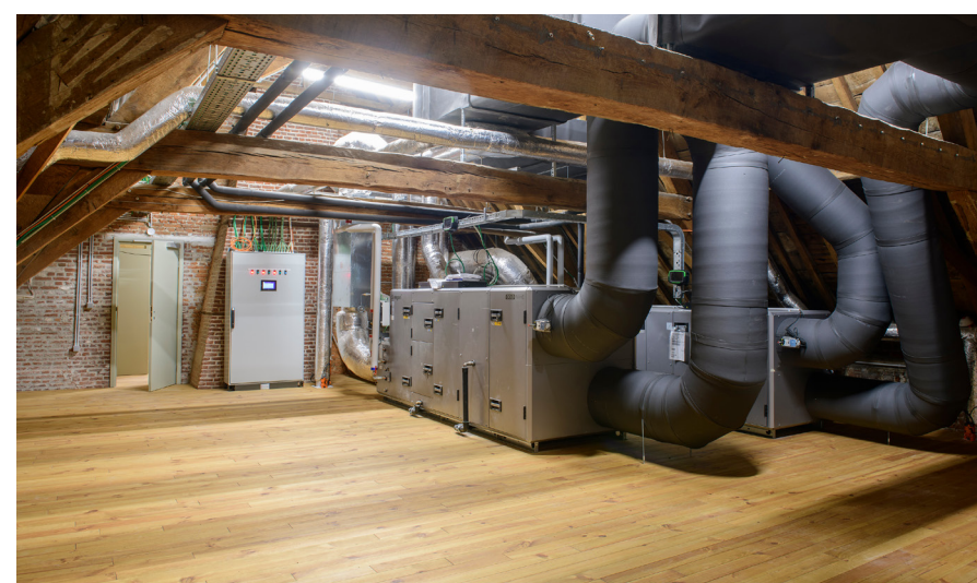
Installation technique au grenier. © Jo Exelmans
